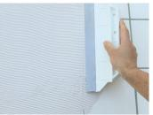
Fit and press pieces tapping well to ensure levelling and good transference of the adhesive.
