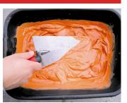
Apply within 3 hours after preparation, spreading the paste over the tiles diagonally using a rubber spatula. Continue until the joints are properly filled.
