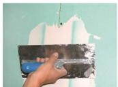
With adhesive netting: bond the netting band to the boards, centring the netting band on the join between the two boards. Apply Tuforte Juntas to the bands. Press well.
