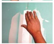
Cover the band again with a new layer of Tuforte Juntas. The mortar to cover the band must leave a thickness of approximately 10 cm to either side. If necessary, repeat the operation. After the Tuforte Juntas has hardened, apply a general layer so as to provide a smooth finish.
