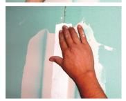
Re-cover the roll with a second coat of Tuforte Aqua Plan. The mortar to re-cover the roll must overlap on both sides by approximately 10 cm.
