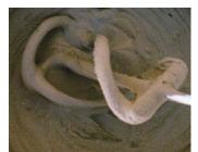
Apply Tuforte Esboço manually with a metal trowel with upward movements, applying two layers until a thickness of 3 mm is obtained.
