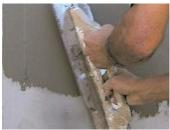
When begin to harden (press the mortar with a finger and does not suffer deformation) proceed to finish sanded using a trowel sponge.
