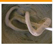
Spread over the support with the aid of a metal trowel or spatula, in thin layers, make up a final thickness of 2 mm, filling and smoothing the surfaces.
