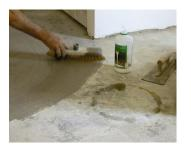
Mix Betonilha Cem mechanically with around 3 litres of water until a smooth and even paste is obtained. The screed should have the consistency of "moist soil".
