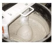
Apply Topeca B-therm directly onto the support. Regulate and / or level the product with aluminum strip to the planned quota. The filling mortar has to be compressed to a smooth surface and without outcrops of water.
