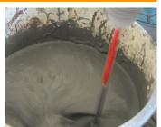
Pour the Autonivelante Nível TOP on the surface to be levelled.
