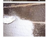
Smooth with an appropriate runner. As soon as mortar Anti-humidade CG starts to harden use a polishing trowel.
