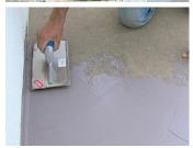
Should you wish to apply a covering to the surface, bonding can be carried out using the same product. Apply Top Elastic K2 using a serrated trowel with teeth which are of a suitable dimension to the thickness of the covering being used. Gently strike the covering to expel any air and ensure full contact.
