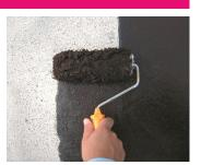
Can be applied with roller, brush or spray gun. Apply  $2^{nd}$  coat after  $1^{st}$  is dry. If necessary apply  $3^{rd}$  coat. Apply using cross coating.
