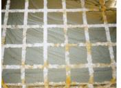
Apply Rebetop Chapisco with projecting equipment in a discontinuous layer, coating only 70 to 80% of the surface and in such a way that it becomes rough.
