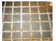
Apply Rebetop Plus Hydro in a single coat, working from bottom to top on the surface. Thickness per layer: 15 - 20mm.
