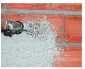
After projecting the paste, smooth out with a cement edger so as to obtain a level surface.
