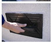
Allow Rebetop Gran to adhere a little then finish with trowel. Wash trowel several times to improve lubrication and facilitate finishing.
