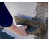
Level out surface passing over with trowel horizontally and vertically until an even layer is obtained.
