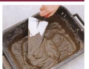
Apply in a regular and continuous thickness. Place elements, compressing and adjusting as required.
