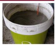
Pour the Topeca Grout over the surface to be filled.
