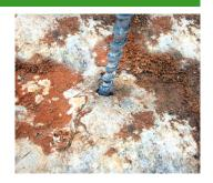
When demolishing objects or structures which are connected to others which are not intended for demolition, it is necessary to create spaces/separation points which allow the expansion of Topeca Dinamit but avoid damage to structures which are to remain intact.
