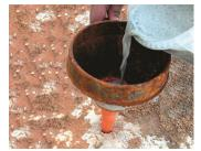
In less than 10 hours Topeca Dinamit produces an expansive pressure of more than 5000 Ton/m<sup>2</sup>. The expansive strength of Topeca Dinamit increases progressively over a period of days.
