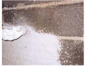
After projecting the paste, smooth out with a cement edger so as to obtain a level surface.
