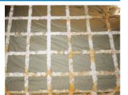
Apply Rebetop Ecolight in a single coat, working from bottom to top on the surface. Thickness per layer: 15 - 20mm.
